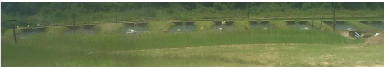
The inlets to the fish ponds from the main river
